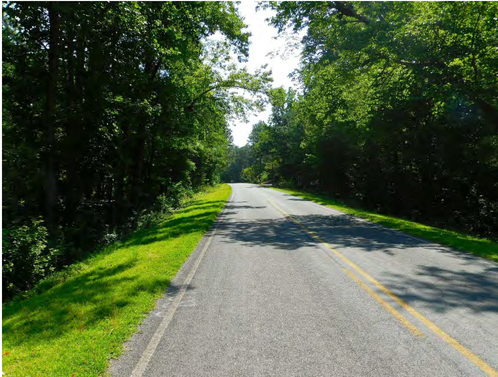
VIEW OF HOLLY GROVE SCHOOL ROAD LOOKING WEST
