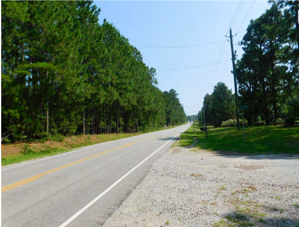
VIEW OF HOFFMAN RD LOOKING NORTH
