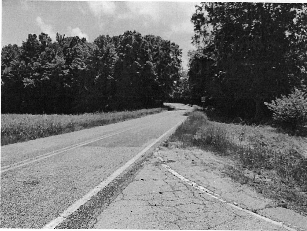
Southbound view West Side Road
