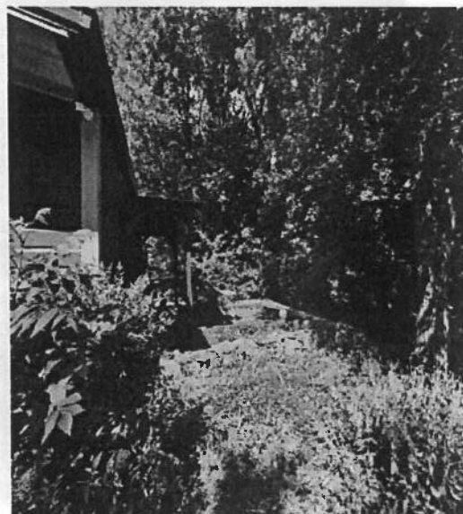
Rear side of 3883 Busbee Road Bldg
