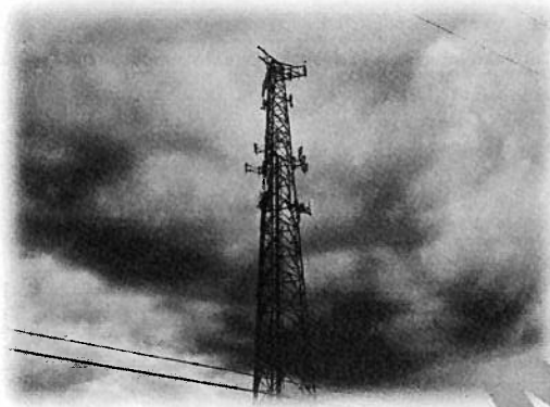
Figure 1.3. Telecommunications Tower. Source: Bing
